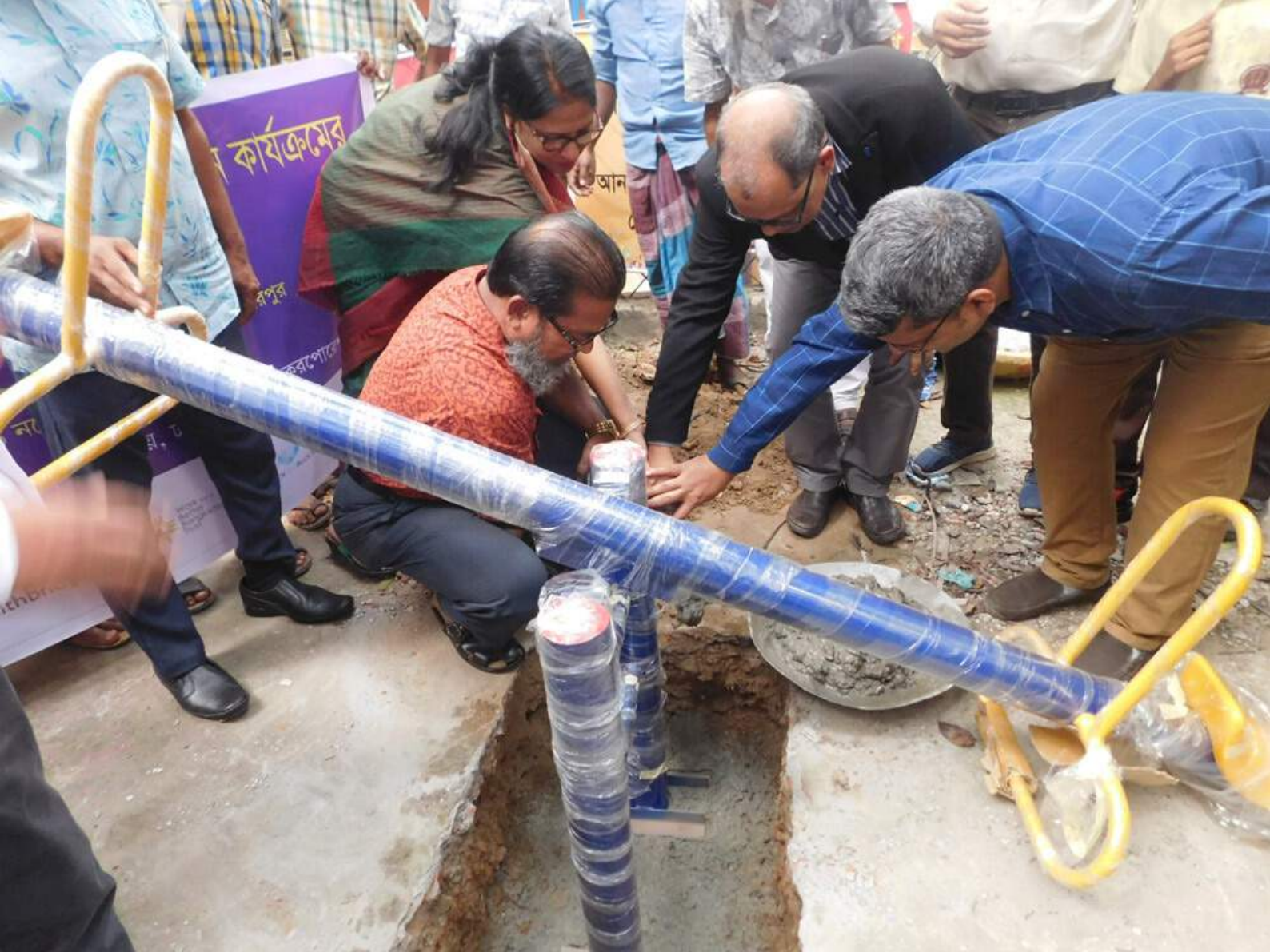
Work opening in ward 2, Pallabi (road 5/6)
